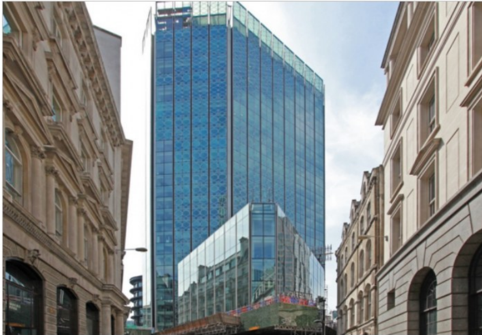
125 Old Broad Street after most recent recladding
